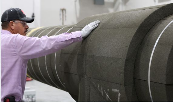
FOAMGLAS® insulation installation.
