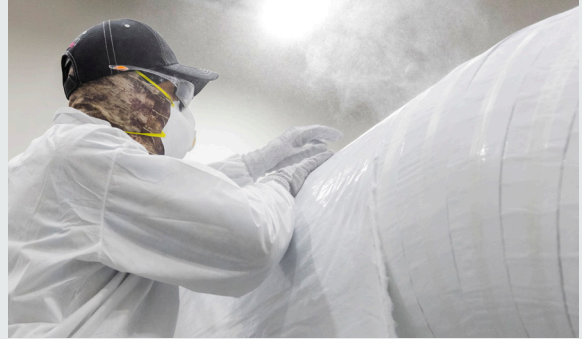
Cold-service aerogel blanket insulation installation.
