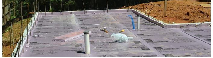
Boards should be installed tightly together.
