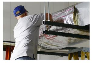
Before applying SOFTR® Duct Wrap, ducts shall be clean, dry and tightly sealed at all joints and seams. Install in accordance with instructions so that compression is controlled.
