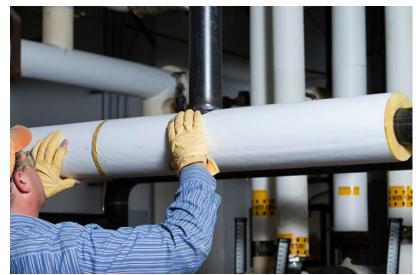
Note: After adhesive tack and when the butt strip is applied, it is critical that the closures are not re-opened and repositioned on the facing. Doing so will diminish the bond strength.
