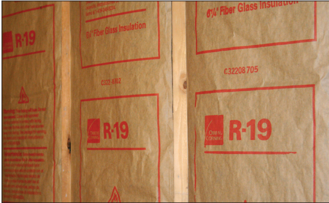
Properly installed faced fiberglass insulation, resulting in a Grade 1 rating.
