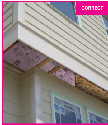
7. CANTILEVERS —Insulate any overhanging floor cavities before closing them in with rigid sheathing (TERC 3.2.2)
