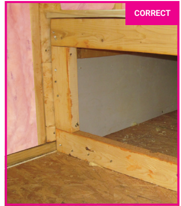
8. TUBS/SHOWERS/FIREPLACES —Insulation is installed behind showers, tubs, and fireplaces on exterior, attic, and party walls and rigid sheathing or other supporting material is installed to hold insulation in place (TERC 2, 3.1)
