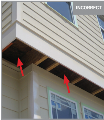
7. CANTILEVERS —Insulate any overhanging floor cavities before closing them in with rigid sheathing (TERC 3.2.2)
