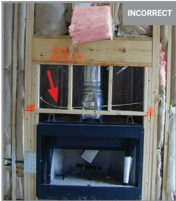
9. TUBS/SHOWERS/FIREPLACES —Insulation is installed behind showers, tubs, and fireplaces on exterior, attic, and party walls and rigid sheathing or other supporting material is installed to hold insulation in place (TERC 2, 3.1)
