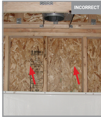
8. TUBS/SHOWERS/FIREPLACES —Insulation is installed behind showers, tubs, and fireplaces on exterior, attic, and party walls and rigid sheathing or other supporting material is installed to hold insulation in place (TERC 2, 3.1)
