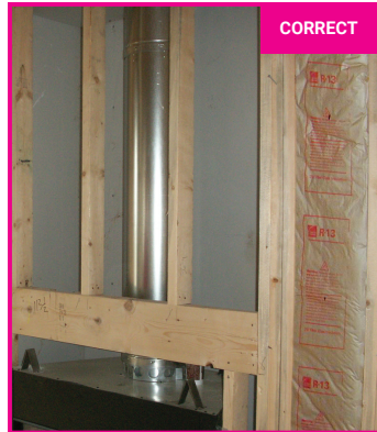
9. TUBS/SHOWERS/FIREPLACES —Insulation is installed behind showers, tubs, and fireplaces on exterior, attic, and party walls and rigid sheathing or other supporting material is installed to hold insulation in place (TERC 2, 3.1)
