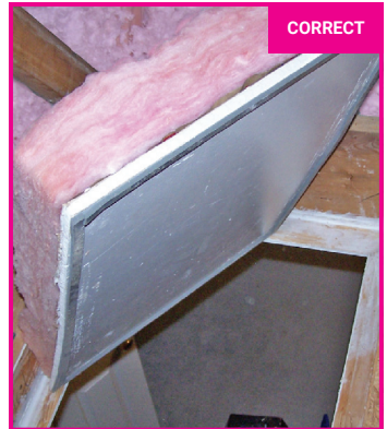
10. ATTIC ACCESS —Access panels to attic/kneewall, drop-down stairs, and whole-house fans are weather stripped and insulated to the same R-value as the surrounding area when possible (min. R-10) (TERC 5.3)
