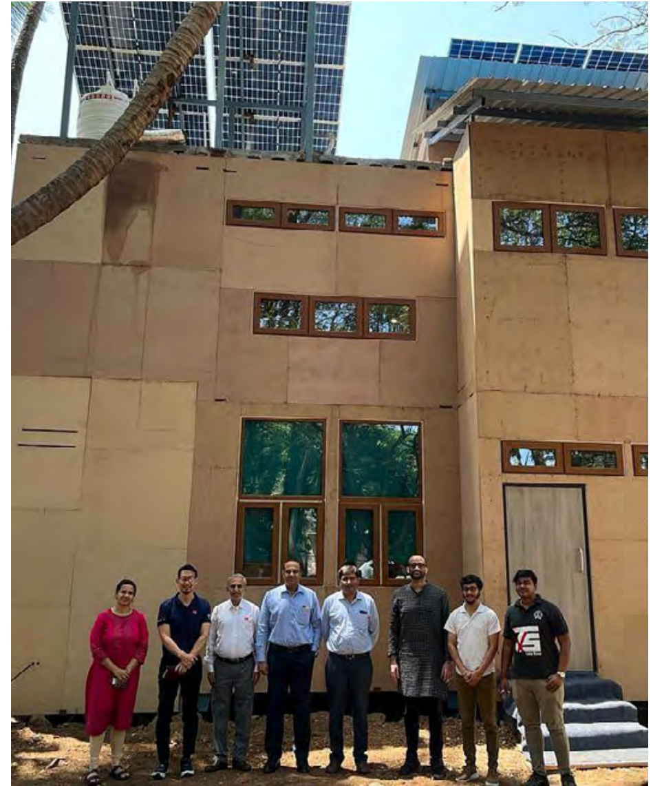
EcoTouch® insulation was used in the construction of this net-zero housing prototype, built on the Indian Institute of Technology campus as part of a competition organized by the National Renewable Energy Laboratory. Paul Wei, Senior Vice President and AP Managing Director, and Dhananjay Tapasvi, India Managing Director, visited the building in April 2023.
