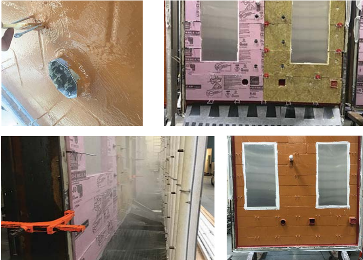
Photos: Penetrated wall during air leakage and water resistance testing
