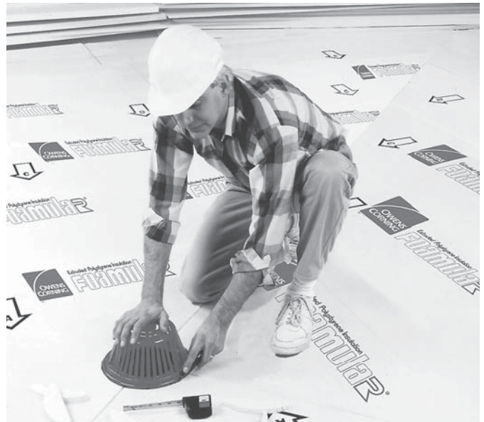
Typical Tapered Roofing Section, 1/8" per foot slope
