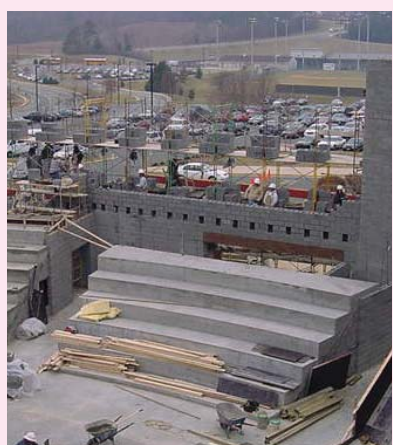
Construction of an 850-seat auditorium at the high school provided an opportunity to test rigid foam insulation placed in service nearly 10 years before.
